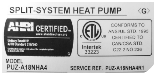
Figure 2: Example of a heat pump nameplate.
