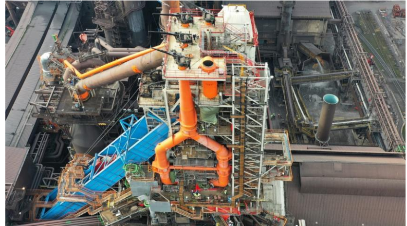
Arcelor Mittal CCUS Pilot Plant in Belgium
